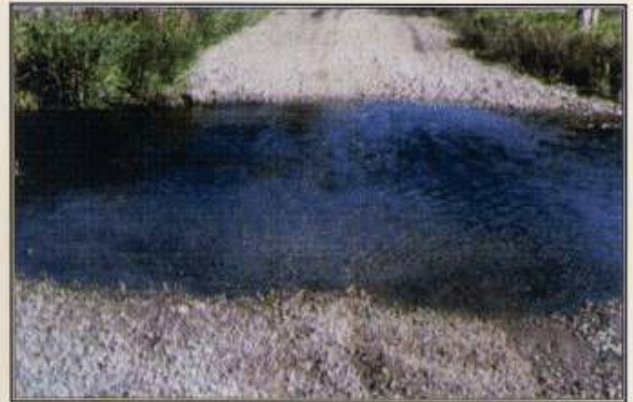
Gravel is used to stabilize this stream crossing.
