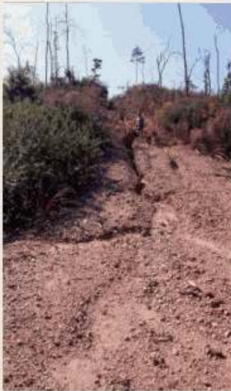
Erosion can be the result of too-steep firebreaks.
